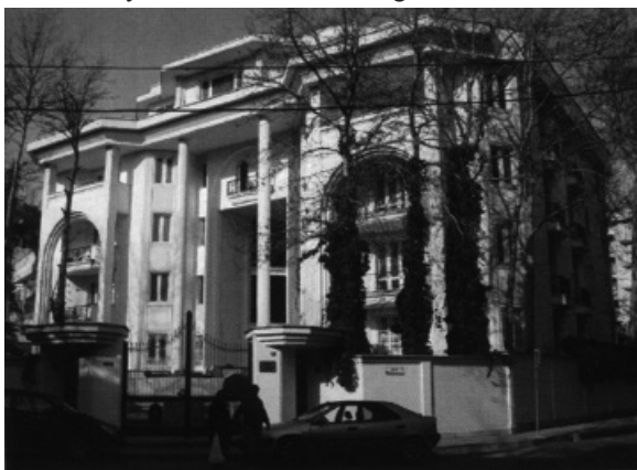
Fig. 1. An image of a good style for architecture, chosen by contemporary Iranian people. (Sadegh Zadeh, 2013, p. 48)
