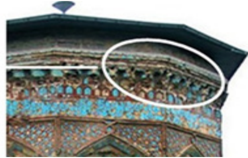
Fig. 8. Maraqa's Kabud Dome
