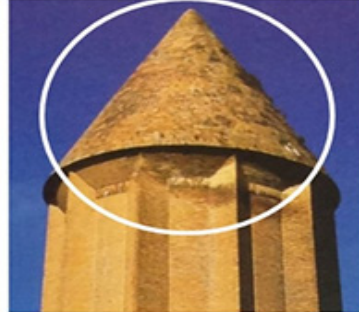
Fig. 2. Kavus Dome and its Spire Vault (Bozorgnia, 2007)
