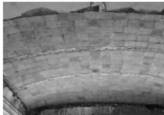
Fig. 4, 5. In Kashan and Tehran , houses the belts are clearly evident in the Lapoosh vaults (Source: The document centre archive of the architecture faculty of Shahid Beheshti University and the paper “Above the Geometry of Vault and Dome”).
