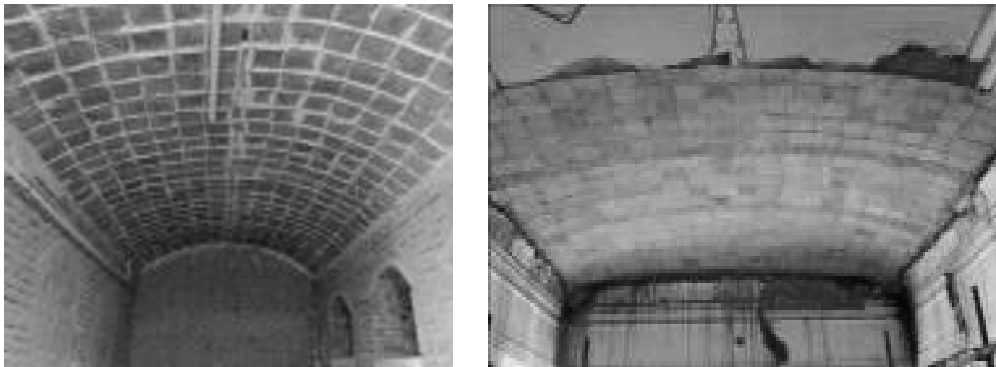
Fig. 9, 10. Two vaults built by the Lapoosh method.
