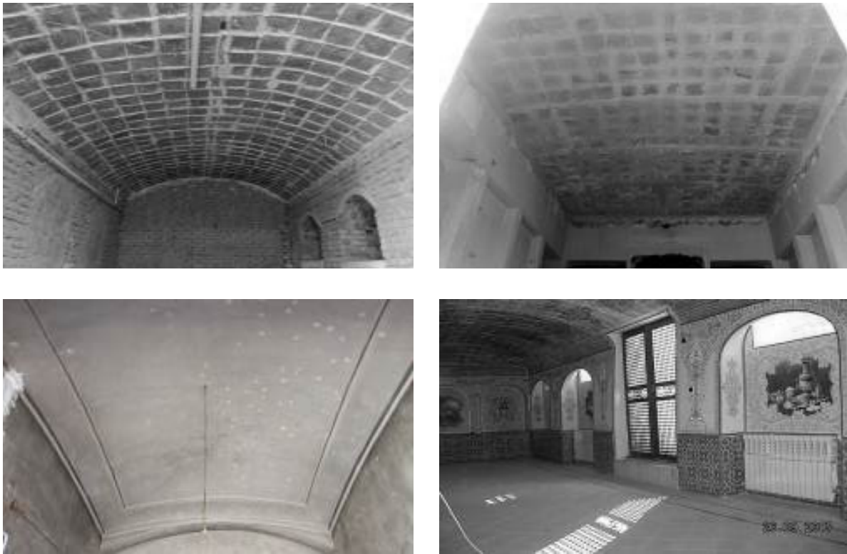
Fig. 16. A few Qomi-poosh vault samples with different deflection (Source: architect Helli's personal archive).
