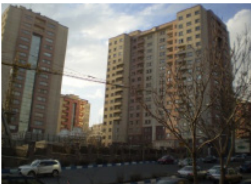
Fig. 4. Tall Buildings without Designed Crown in Tehran.
