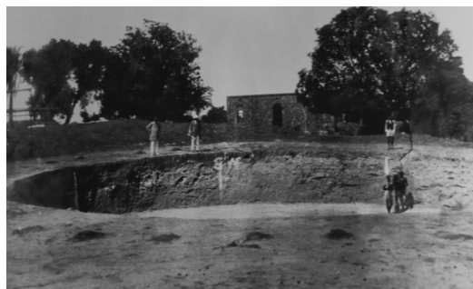
Fig. 2. A Circular Pit is Dug to Prepare for the Construction of Dakhma (Salsette Dakhma of India and Andohen)
