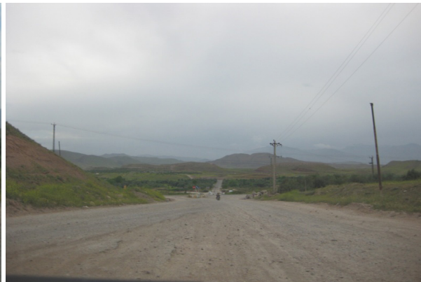
Fig. 6. Loshan's Highway Exit
