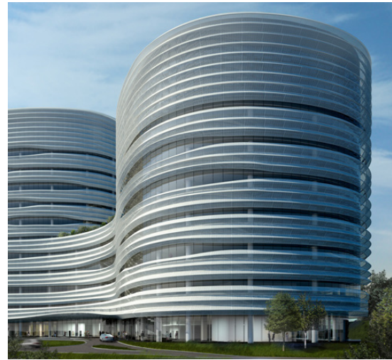
Fig. 9. CJ Cheiljedang Research and Development Center, by Yazdani Studio / Cannon Design. The Foldable Facade Wraps the Whole Building in Ribbons, and is Sectioned Such that Pockets Can be Opened and Closed Where Needed, Picture Taken from (Yazdani Studio, 2011).
