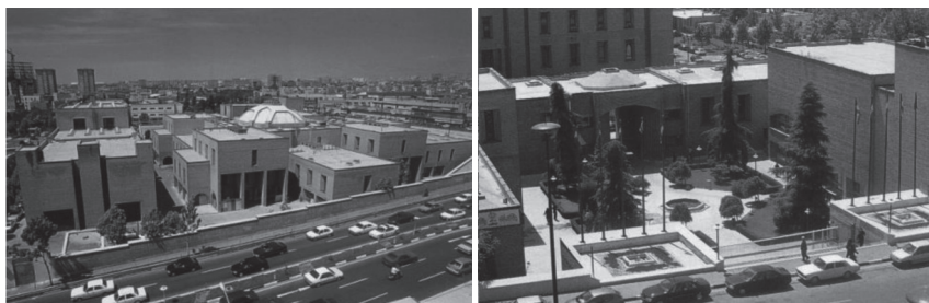
Fig. 14, 15. Central Building of ICHTO (Naghsh, 2008)
