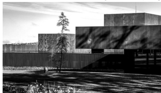
Fig. 12. The Effect of Time (Rust) on the Final Covering of a Building, Soulagés Museum
