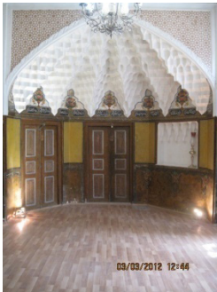
Fig. 1. Muqarnas, Architecture Elements in the Ebrahimi House
