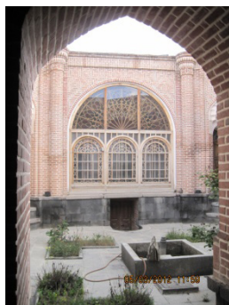
Fig. 10. Exterior View of the Ershadi House
