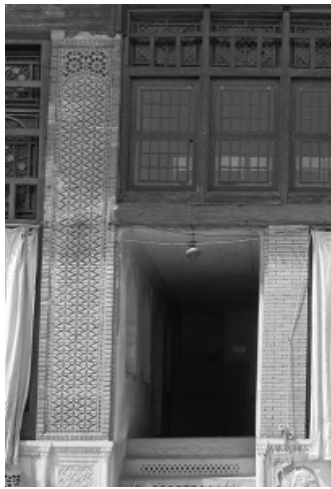
Fig. 8. Walls on Sides of the Main Hall are Covered with Tiles (Left) While others are not (Right)
