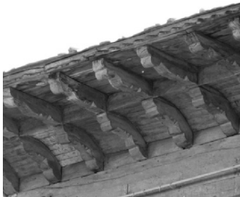
Fig. 13. A Longer Double Stepped Shirsari in the West Side of Zinat House
