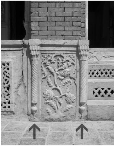
Fig. 7. Representational Figures of Columns in Decoration- The Designer has Tried to Indirectly Show the Presence of a Structural Wall (Representational Tectonics)
