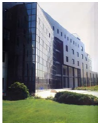
Fig. 19. Telecommunication Center of Yusifabad (Hosseinzadeh & Qolinezhad, 2010)
