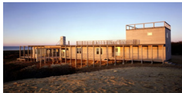
Fig. 10. A Total View of the House (Steven Holl, 2016)
