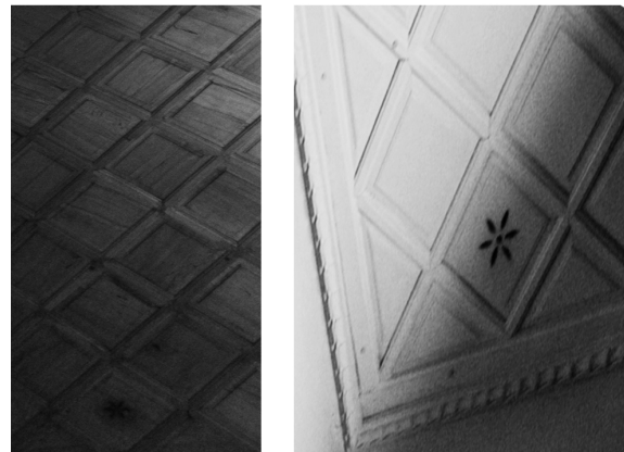
Fig. 16. Lambekubi Ceiling in Two Rooms of Qavam Building
