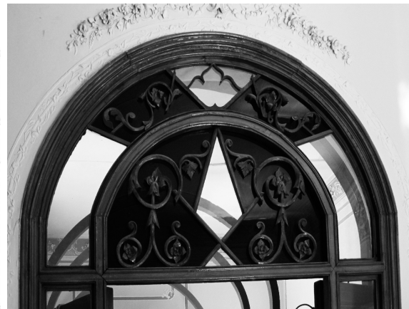
Fig. 14. Windows of Exterior Views at Qavam Building
