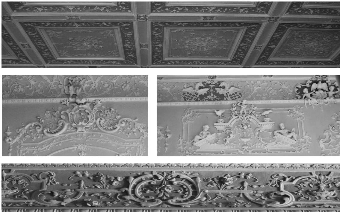
Fig. 11. Trimmings of Qavam Building Ceiling and Walls
