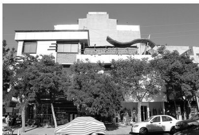
Fig. 10. Lack of Harmony in the Walls of Street
