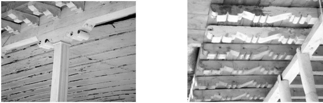
Fig. 5. Decorations Under the Roof of Avansian's House in Rasht: Lathed Cymatium Motifs of the Beams Under the Roof and Motifs of Capitals
