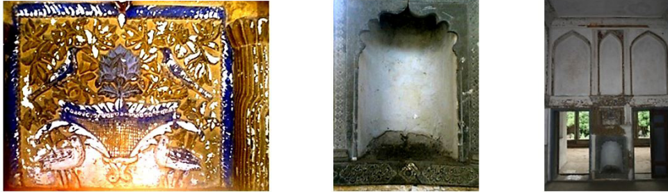
Fig. 24. Location of the Heating System and Plastering of the Upper Part
