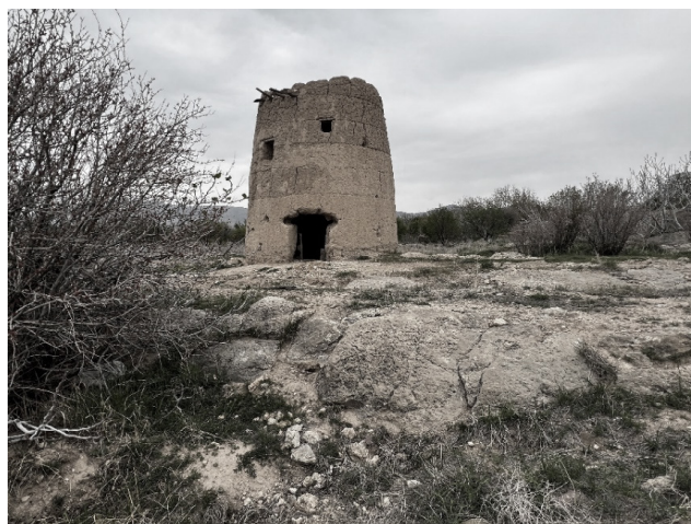
Figure 13: The entrance door to the Rezaabad watch tower
