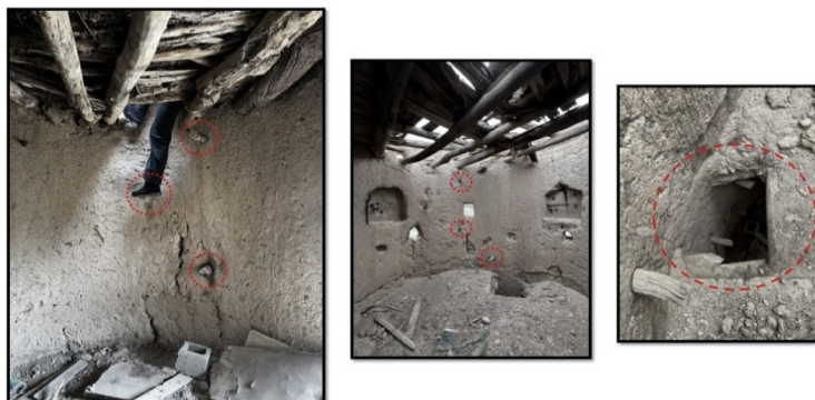
Figure 12: How to access the first floor, case of Rezaabad watch tower
